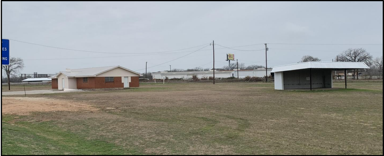
2200 Air Base Road Freewill Church (During)
